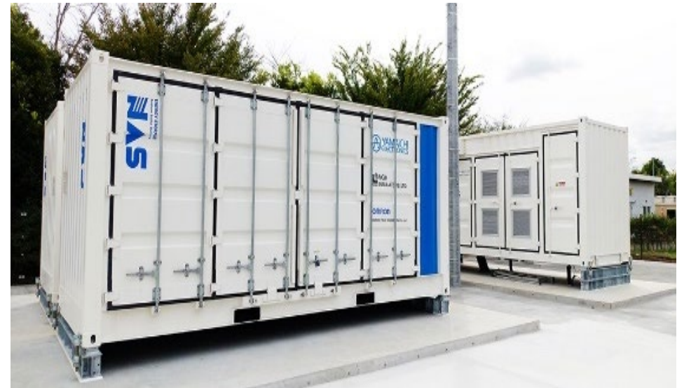
Sakura Factory's NAS battery system: Capacity 2,400 kWh/Output 400 kW
